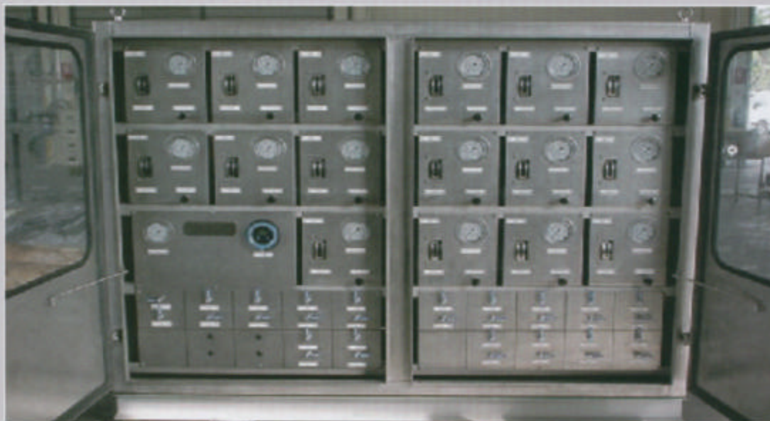
Typical Haskell IRCD panel injecting chemical into 16 injection points, utilizing only one small pump and one spare. Note the apparent ease of operation and layout.
