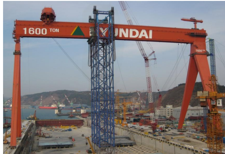
Crane Lifting 5,800ton(Ulsan)
