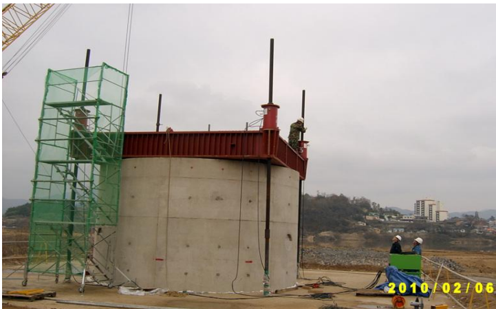
Well inserting operation
