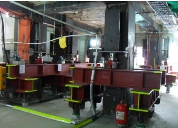
Job site installing
