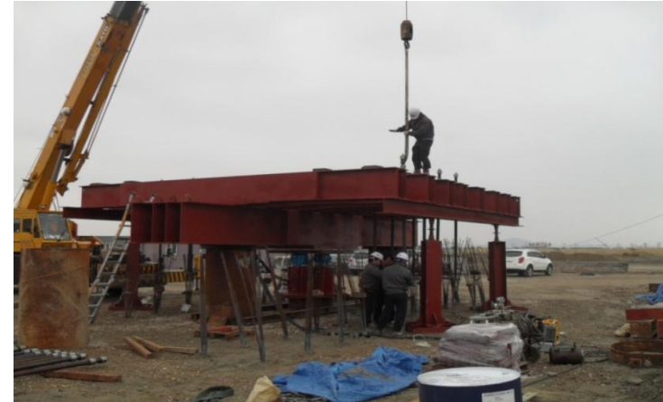
Compression load test at the top
