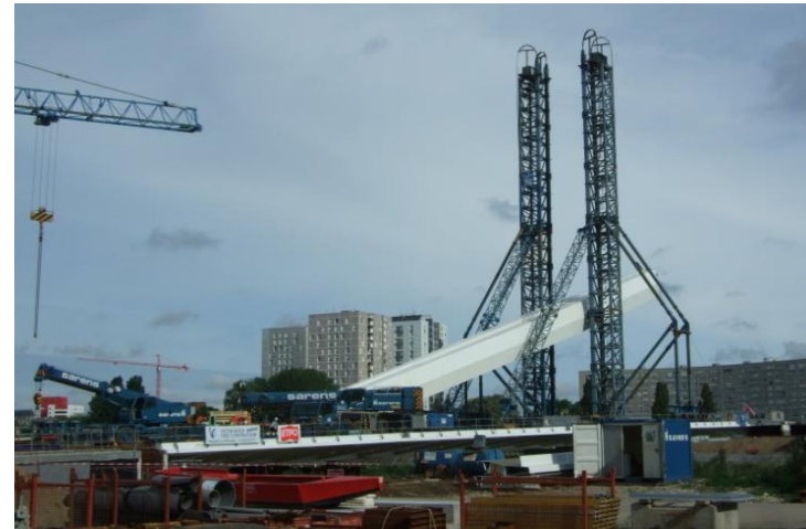
Vertical lift(France) Strand Jacks 8x200ton
