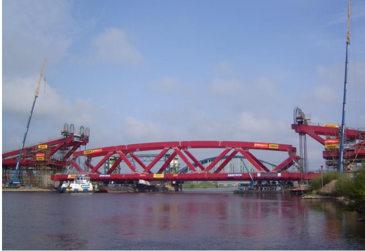
Bridge Lifting 2,500ton(Netherland) Strand Jacks 8x450ton
