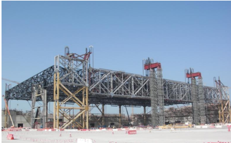
Roof Lifting 10,500ton & 9,500ton (Qatar Doha) Strand Jacks 20x450ton + 8x650ton + 4x200ton
