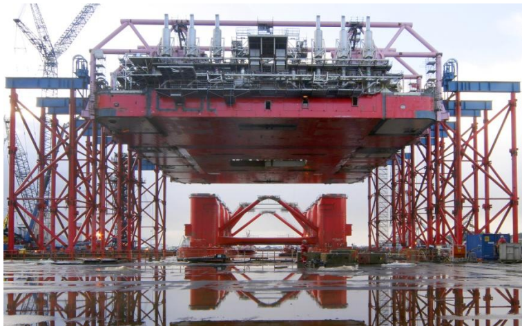
Drilling Rig 10,700ton & 9,500ton (Norway) Strand Jacks 32x450ton
