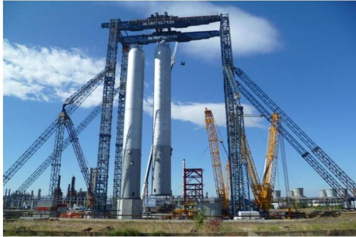
1,400ton tower lifting
