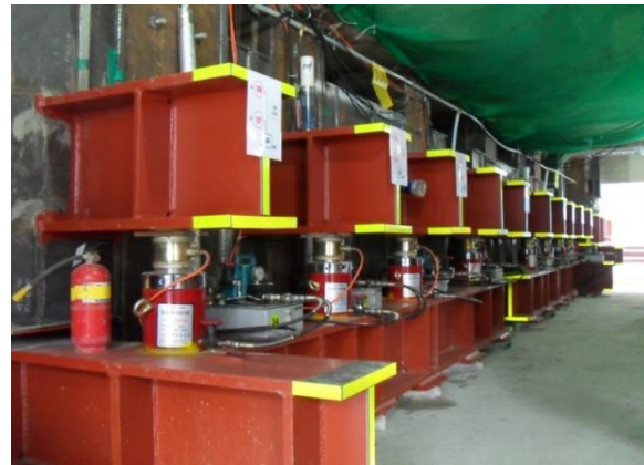
Completion of installation
