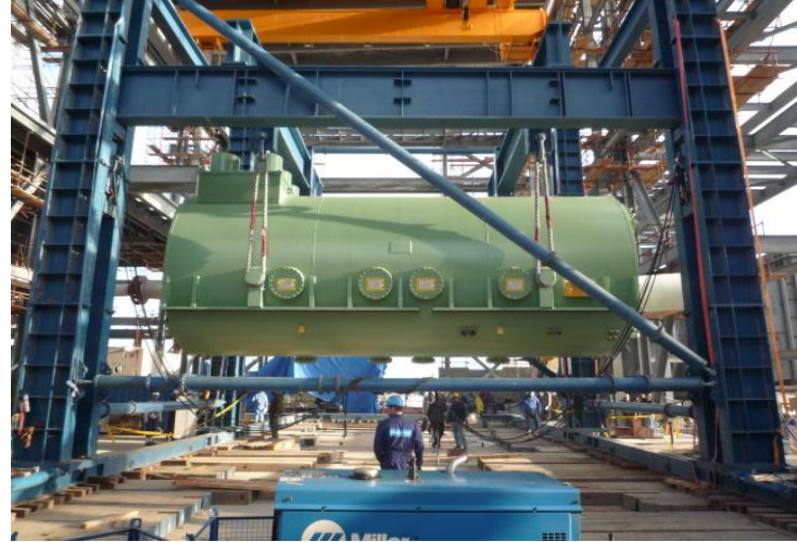
Stator installing
